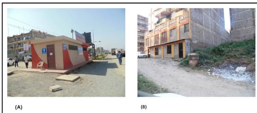
Figure 6: Plate showing (A) a public toilet in Mlolongo (B) sewer line in Ruiru
