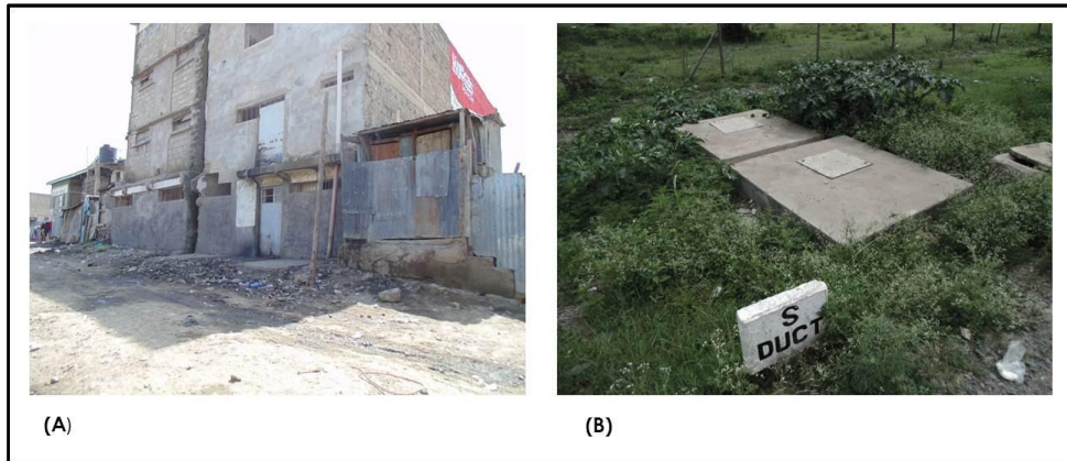
Figure 8: Plate showing (A) community toilet in Mlolongo (B) sewer line in Ruiru
